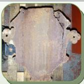
We were contacted by a company who were renovating a Victorian property to repair two cast iron water hoppers which were in need of new spigot sections, and one of them had a large crack to the back face which would need fusion welding.
