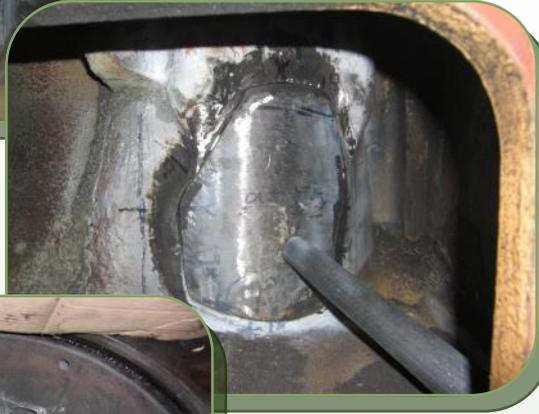
Working throughout the night using our Lock and Pin methods, the patch was carefully stitched into place.
